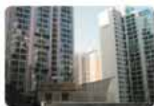
Apartment Expansion Joint
